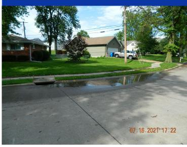
Stormwater runoff from the upper reaches of the drainage area flows south and ponds on a paved patio at 2706 Lakeport Drive and a flat or low-lying area at 2712 Lakeport Drive. There is minor yard rutting evident at the rear southeast corner of the property at 2715 Lakeport Drive. A portion of the surface drainage crosses the public sidewalk and flows onto Lakeport Drive before entering a curb inlet in front of 2712 Lakeport Drive and is considered a nuisance.
